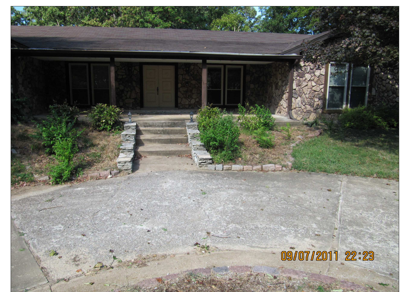
REMOVE AND HAUL EXISTING SOD IN PLANTED AREAS ON EA. SIDE OF STEPS. SALVAGE COBBLESTONES FOR REUSE. INVESTIGATE ELECTRIC LINE AND SOURCE PRIOR TO PLANTING
